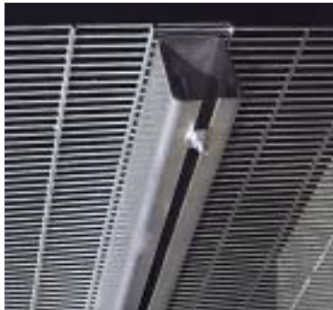
WELDED MESH "C" POST OVERLAP
